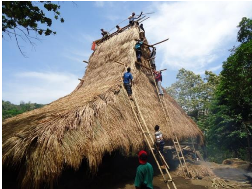
Fig. 9. Topping-off the highest part of Sao Ria Source: Author's Documentation, 2014.
