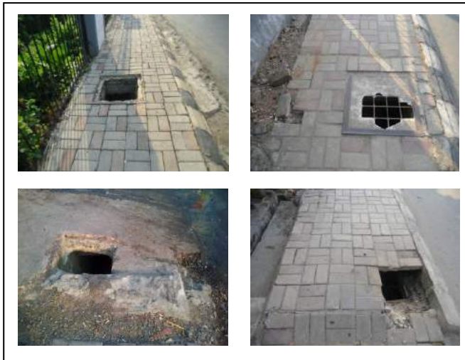
Figure 8. Drainage Hole Condition Source: Author
