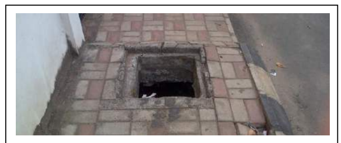
Figure 3. Drainage Hole Source: Author
