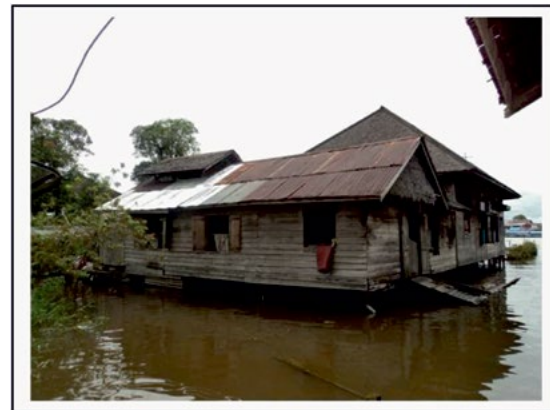
Figure 8. The flood conditions in the town of Tayan due to the upstream overflow of Kapuas river. According to information, overflow of the river water will flood the land at least for a week and this was routinely occurring throughout the year (the photo was taken at December 2010 from the rear side of the case on Tayan town).(Author, 2012)
