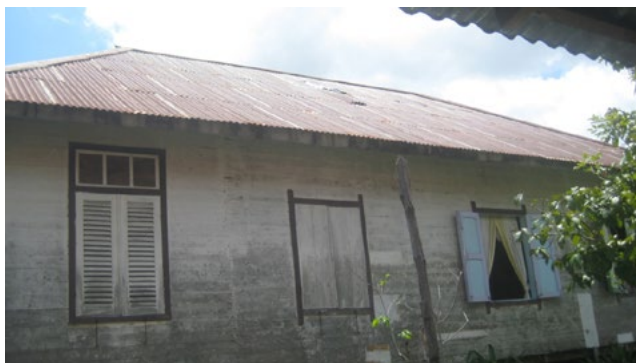
Figure 5: House elements was designed to suit the local climatic requirements using various ventilation and solar control devices and low thermal capacity building materials (the photo was taken on December 2010 from the rear side of the case on Sambas town).
