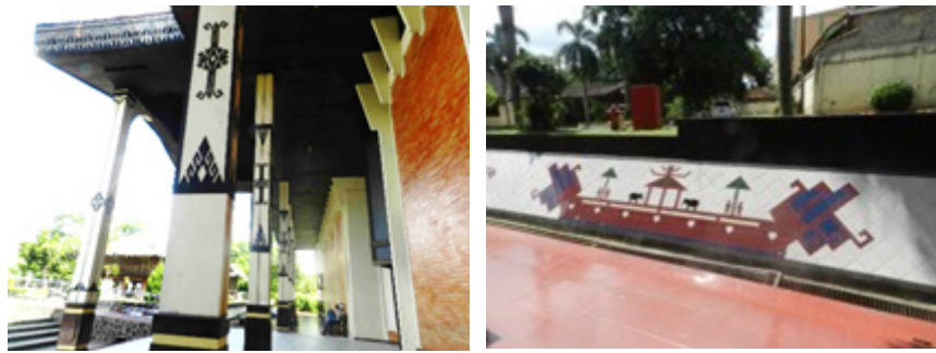
Figure 2 the building ornament (Clara, 2016)
