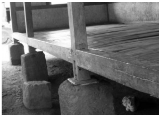
Gambar 4. pondasi umpak
