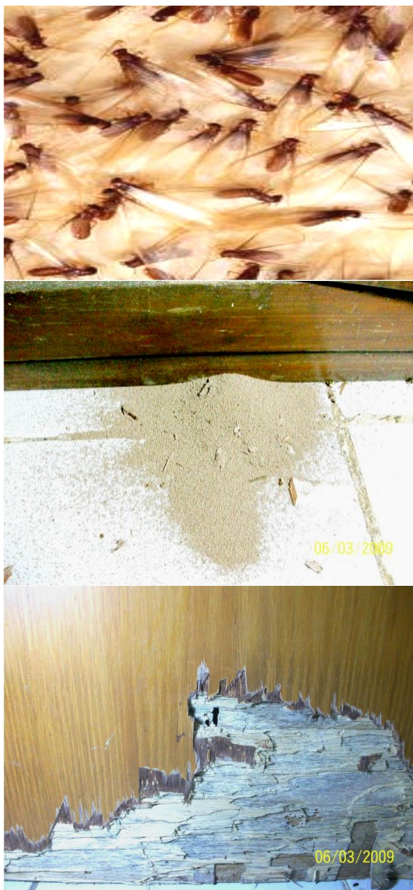
Figure 3. Signs of termite infestation: Adult died and discard wings ( top ), fecal pellet ( centre ), and damage wood ( bottom )
