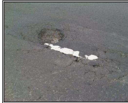
Gambar 3. lubang (*potholes*)
