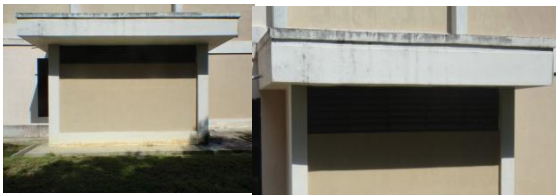
Figure 3. Experimental building with concrete roof Source: Private documentation, 2011
