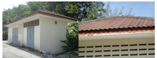
Figure 1. Experimental building with ceramic roof Source: Private documentation, 2011
