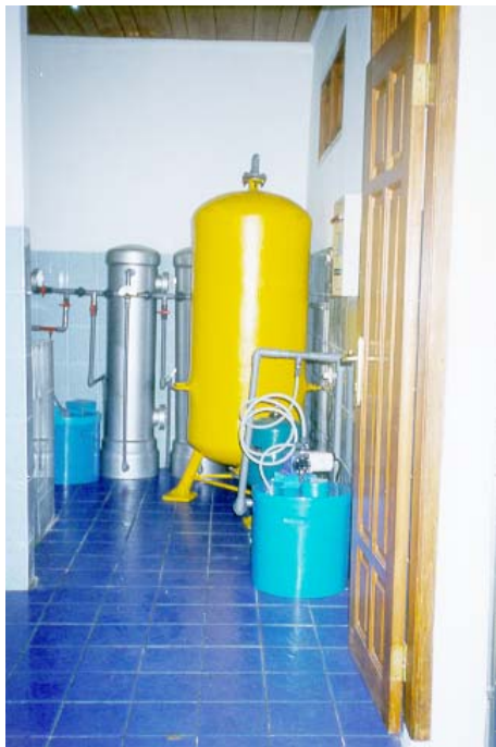
Gambar-8 Chemical tank, pompa air baku, mixer, dosing pump, reaktor tank dan Instalasi Filter
