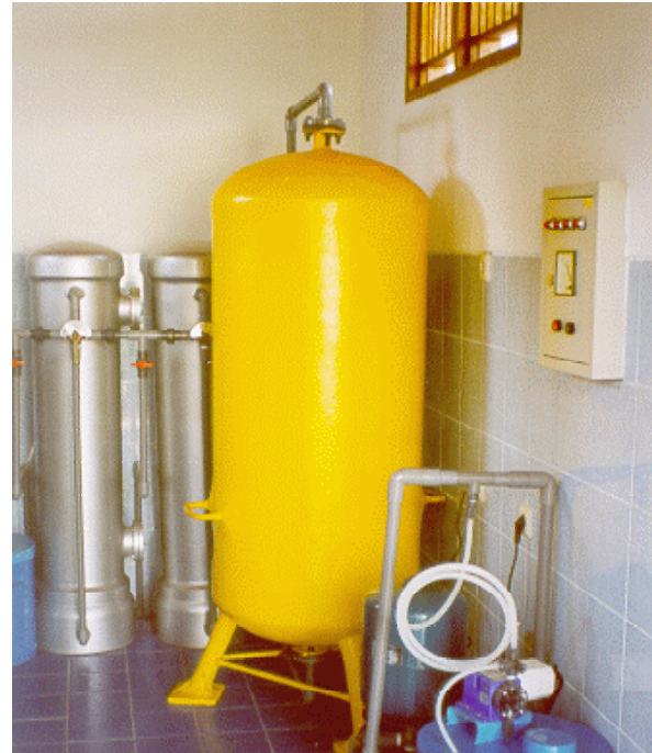
Gambar-8 Chemical tank, pompa air baku, mixer, dosing pump, reaktor tank dan Instalasi Filter
