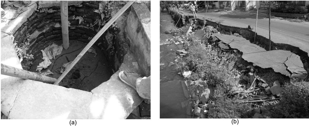
**Figure 1. Liquefaction phenomena found in Yogyakarta 2006 (a) sand boiling in an open well (Adi, 2013) (b) lateral spreading on edge state road (Adi, 2013)**
