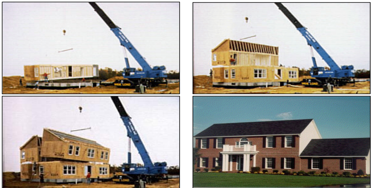
Figure 1. Typical erection of modular home (source : Building System Council, USA)
