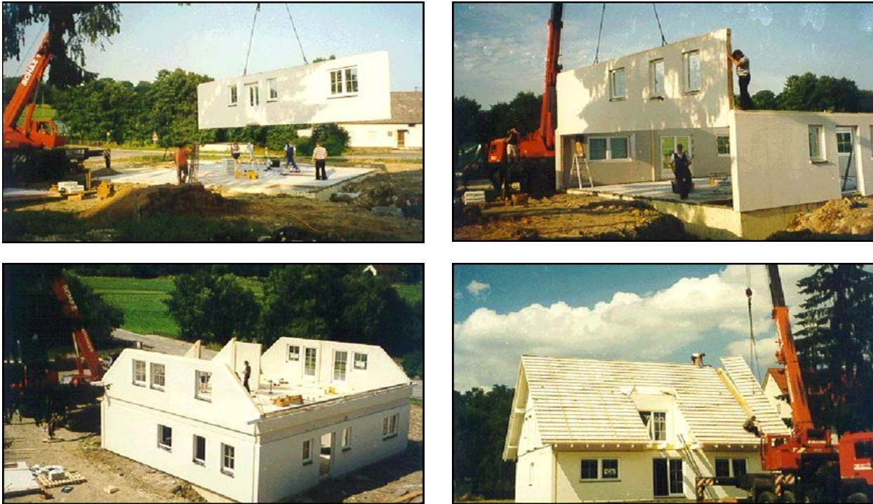
Figure 2. Typical erection of panelized home (source : Bodenhaus, Germany)
