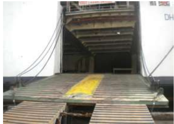
Gambar 4.1 Tampak depan side ramp door KM. DHARMA KENCANA II
