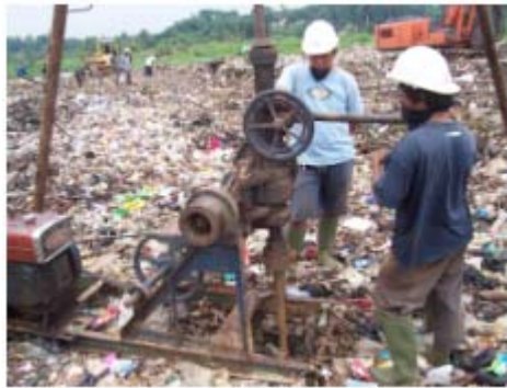
Figure 3. Picture of boring activity for inserting gas venting pipe.
