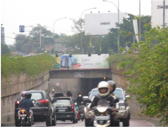
Figure 2 View of the Underpass Taken from Simprug
