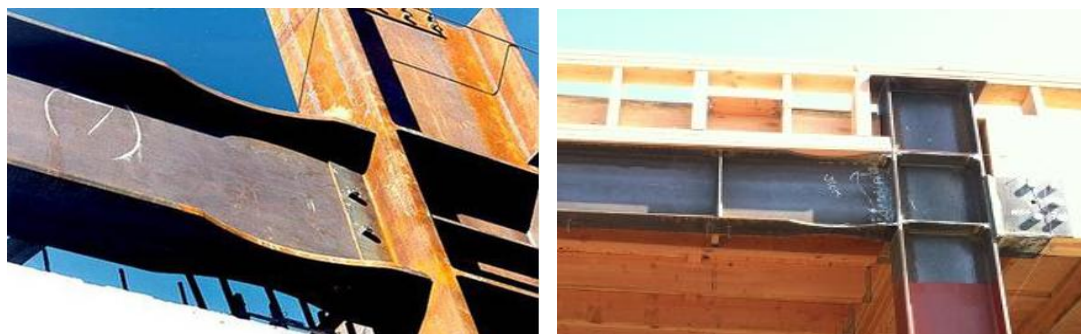
Figure 2. Application of Reduced Beam Section (RBS) Connection
