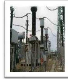
Gambar 6. Tranformator Tegangan
