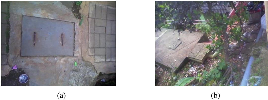
Figure 3. The condition of: (a) Inspection chamber no.2; (b) inlet of the septic tank
