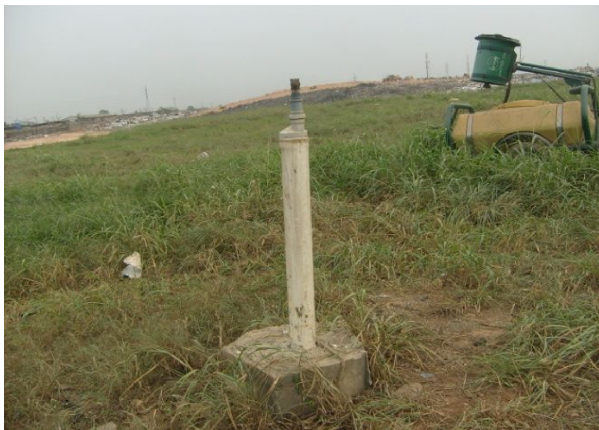
Figure 6. A well-head for LFG capture at Olusosun
