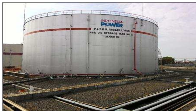
Gambar 1. HSD Oil Storage Tank
