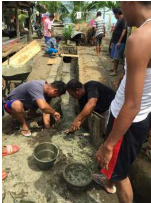
Gambar 6. Pengecoran dinding drainase
